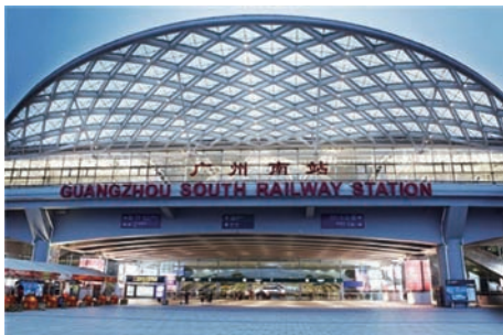
Guangzhou South Railway Station
