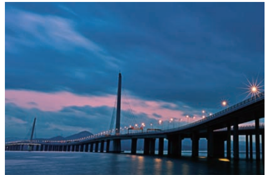
Hong Kong-Shenzhen Western Corridor
